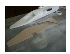
34. Use a hack saw blade to cut a groove for the vertical fin. Adjust the slot as you did for the landing gear plate. Then epoxy the vertical stab in place.
